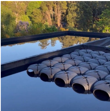
Figure 1: rainwater reservoir formed under Cupolex domes to be employed on the green roof
